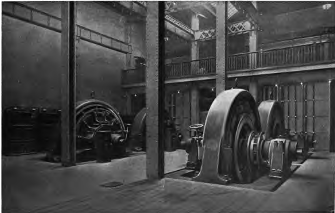
INTERIOR OF SUB-STATION NO. 11
